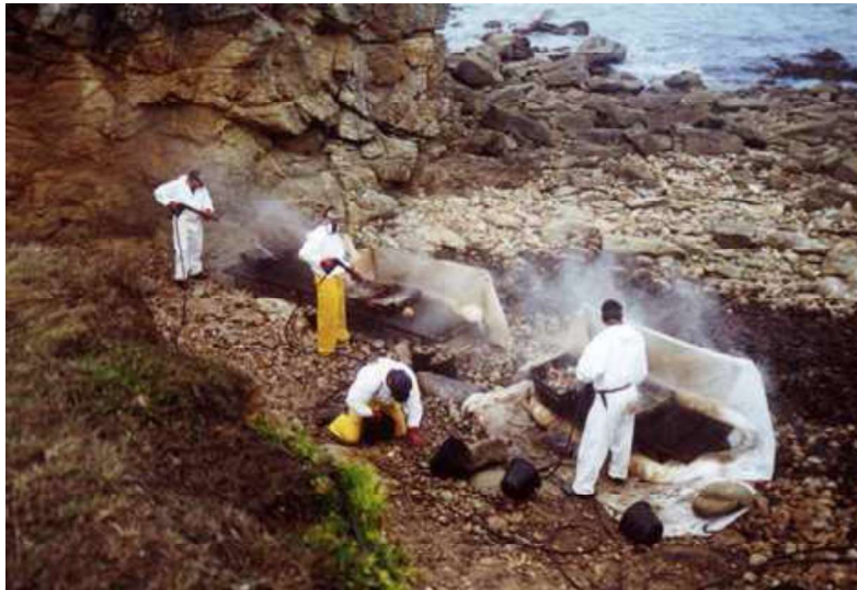
Washing of pebbles on site (Source: Cedre)
