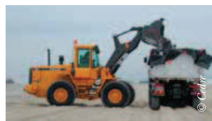
Truck and skip protected with plastic liner
