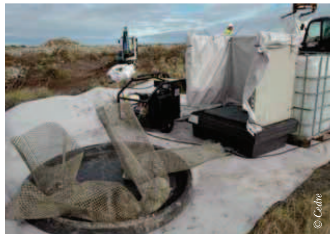
Washing pebbles on site in a booth
