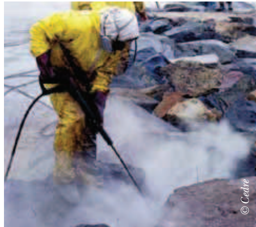
Risks of pollutant splashing
