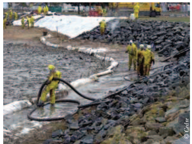
Mechanical clean-up of riprap
