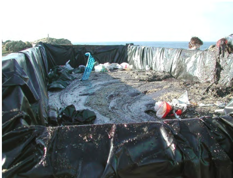
Badly sorted OSW: Semi-solids mixed with some solid waste (Source: Cedre)
