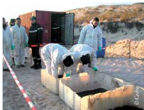
Successive tanks for rough and intermediate cleaning
